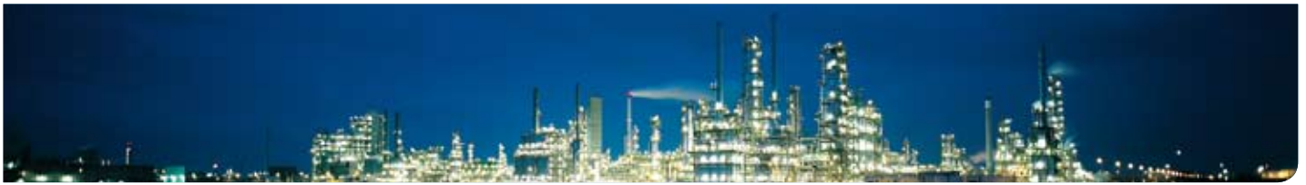
TOTAL Refinery in Central Germany in Leuna
