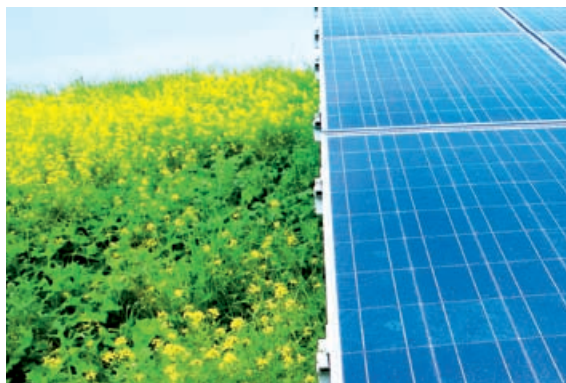
Solar field in Solar Valley
